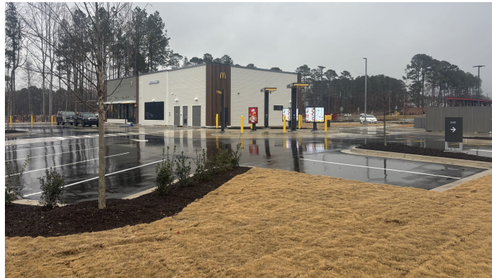
The completed new restaurant at Buffaloe Rd, Raleigh, NC
